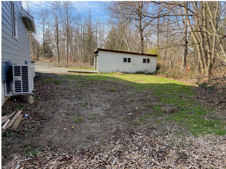
Photo 10. View west along the north side of the house (3/3/21).
